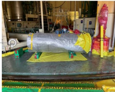
Disassembly of Duct Risers
