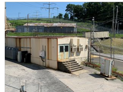
U3 Access Trailer Prior to Start
