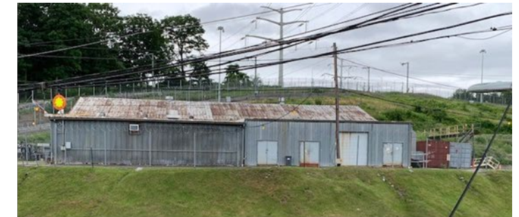
Fab Shop Demolition Prior to Start
